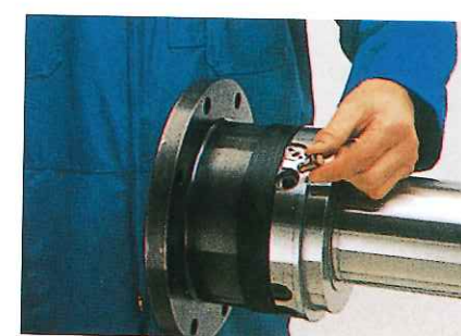
(Step 1) Replace the broken shear tube.
